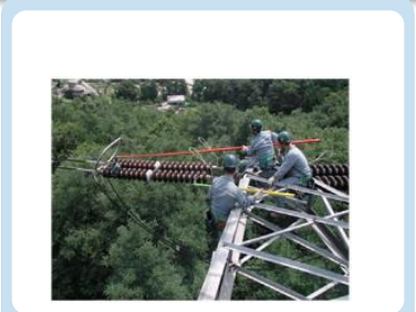
Insulator inspection work using electric field formula detector
